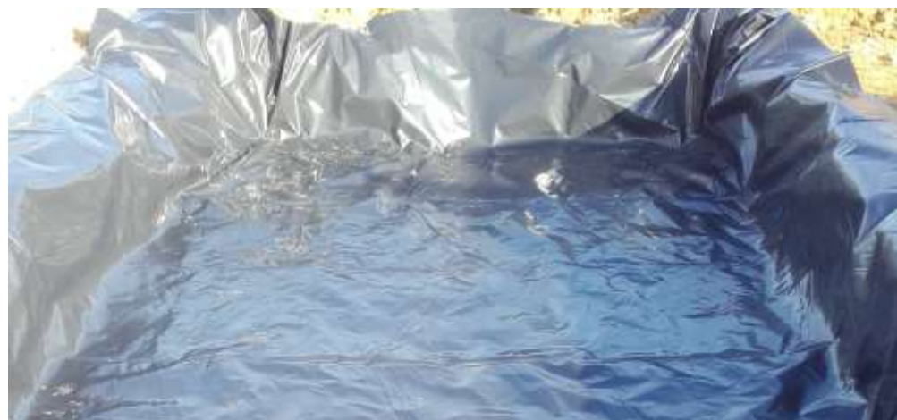
Figure 23 – Installation de la membrane souple
